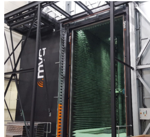
Fig. 4a & 4b - Sliding Door with Associated Supporting Steelwork
