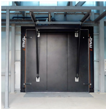
Fig. 4a & 4b - Sliding Door with Associated Supporting Steelwork
