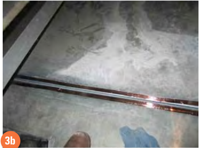
Figure 3. Condition of panel joint at top of chamber. (a) Corrosion on the top of the chamber due to pooled water. The corrosion extends to one of the panel joints. (b) Copper tape was used to bridge between the joint and the chamber panel after corrosion was cleaned away. Corrosion under the joint could not be cleaned.
